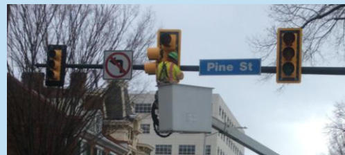
Upgrading 8” to 12” signal heads
