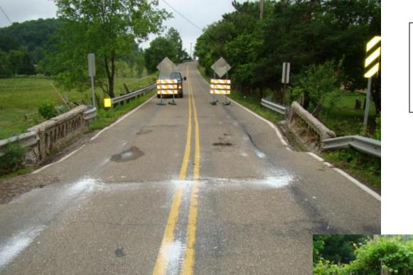
This top photograph shows settlement distress in the roadway due to tilt damage of the abutment.
