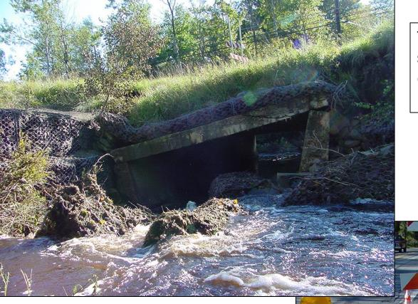
This top photograph shows settlement damage in the abutment due to scour taking away the earth underneath the abutment.
