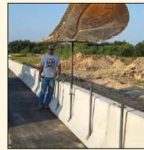
Threaded removable pin extension used for installation & removal
