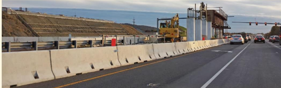
Crash Test Installation photos
