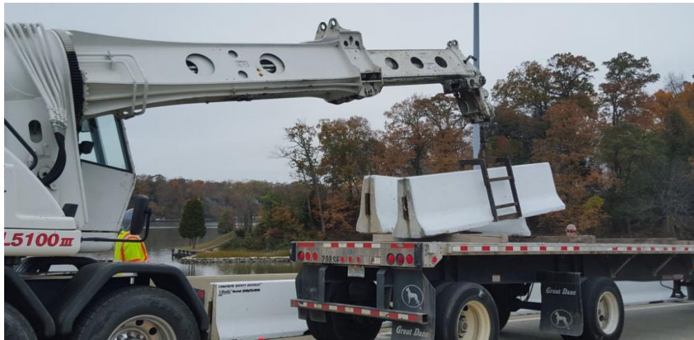
UNLOADING BARRIER FROM TRAILER
