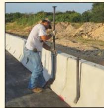
Threaded removable pin extension used for installation & removal
