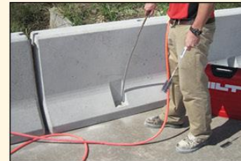
Cleaning hole with air and brushing
