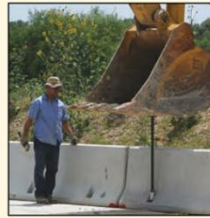
Pins installed - 3 minutes each
