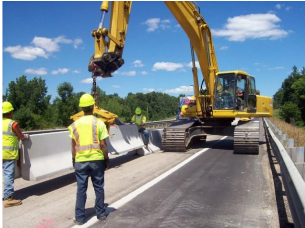
BACKHOE IN USE
